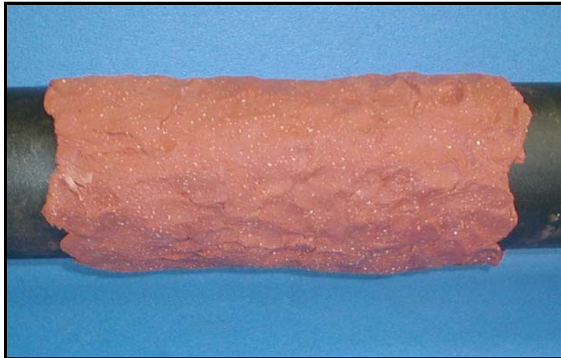
Figure 2-8: Spreading DMP-3 Damping Material
