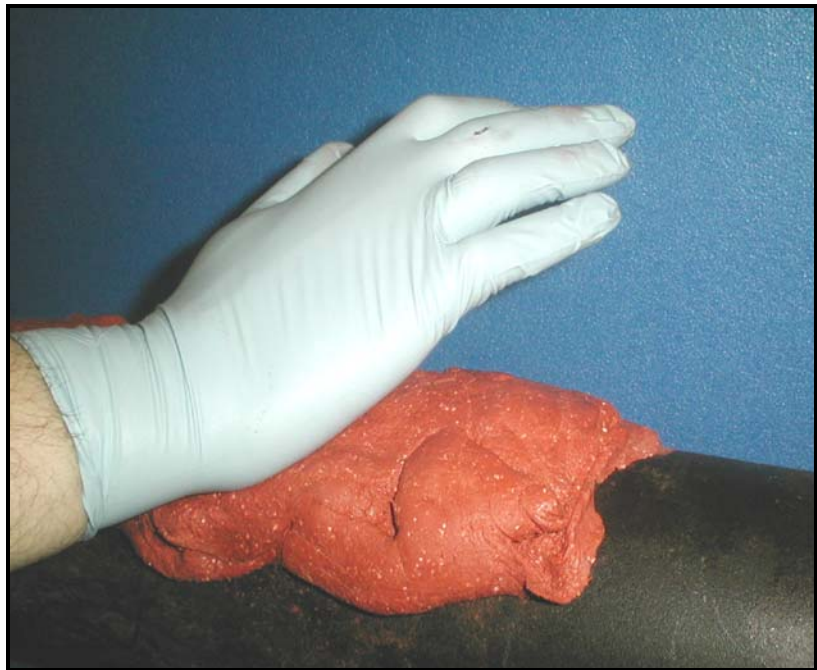
Figure 2-7: Applying DMP-3 Damping Material
